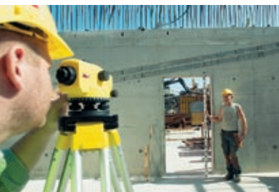
Building and Civil Engineering
